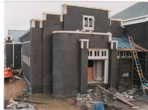
New church hall nearing completion 1997 (top).
